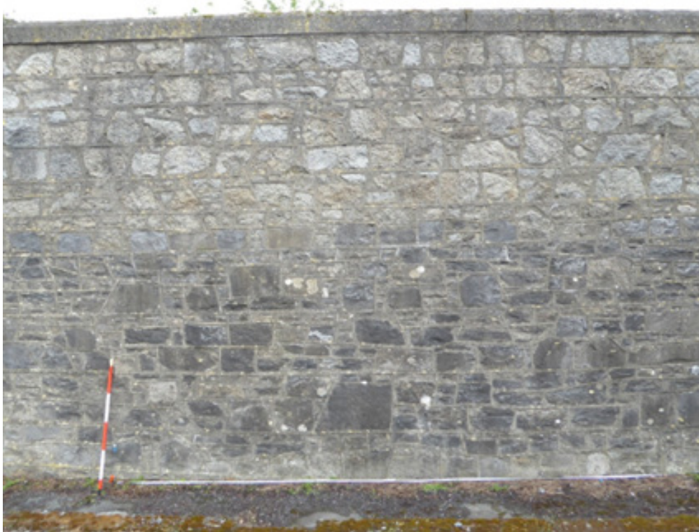
Typical section of walling
