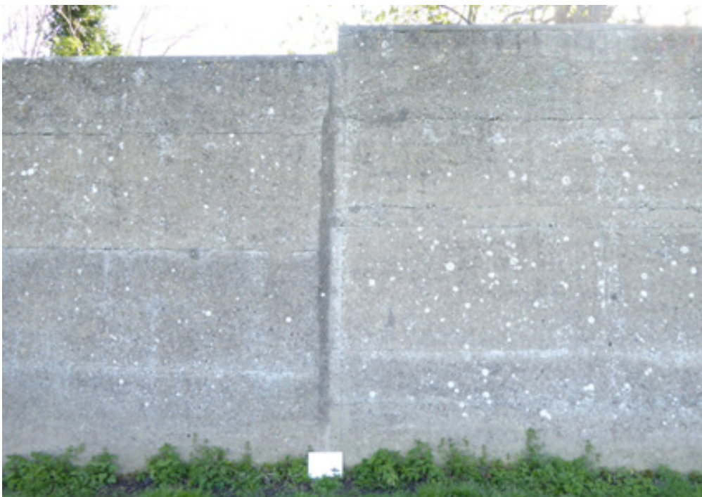
Section of wall comprising in-situ mass concrete
